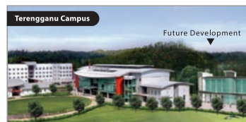
Terengganu Campus Future Development Bukit Khor, PT 11065, Mukim Rusila, 21600 Marang, Terengganu, Malaysia. Tel (609) 628 1880 / 1889 Fax (609) 628 1885 (KPT/JPT/DFT/US/T01)
